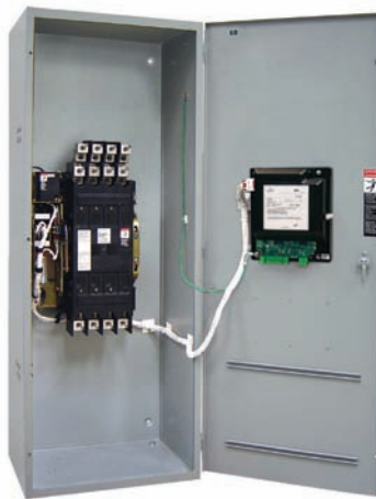
Fig. 4: ASCO Power Transfer Switch rated 600 Amperes
