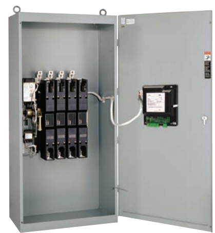
Fig. 5: ASCO Power Transfer Switch rated 1000 amperes
