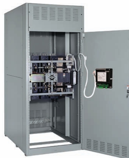
Fig. 7: ASCO Power Transfer Switch rated 3000 amperes
