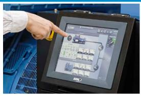
The new APM802 command/control system is specifically designed for operating and monitoring power plants for markets including hospitals, data centres, banks, the oil and gas sector, industries, IPP, rental and mining. This unit is available as standard on all generating sets from 275 Kva designed for coupling. It is optional on the rest of
